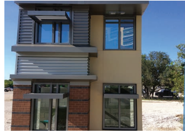
Exterior mock-up for the new Barshop Institute for Longevity and Aging Studies at the University of Texas Health Science Center at San Antonio
