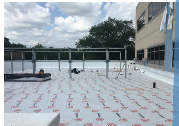
Roof installation at Houston Methodist Willowbrook Hospital, Ambulatory Surgery Center Expansion
