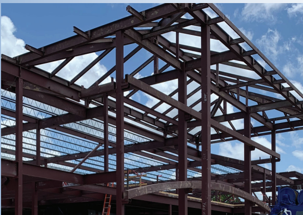
Steel structure for the City of College Station, New Police Department
