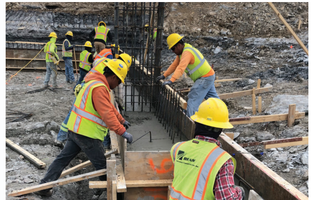
Concrete trade contractors at the Collin College, Celina Campus
